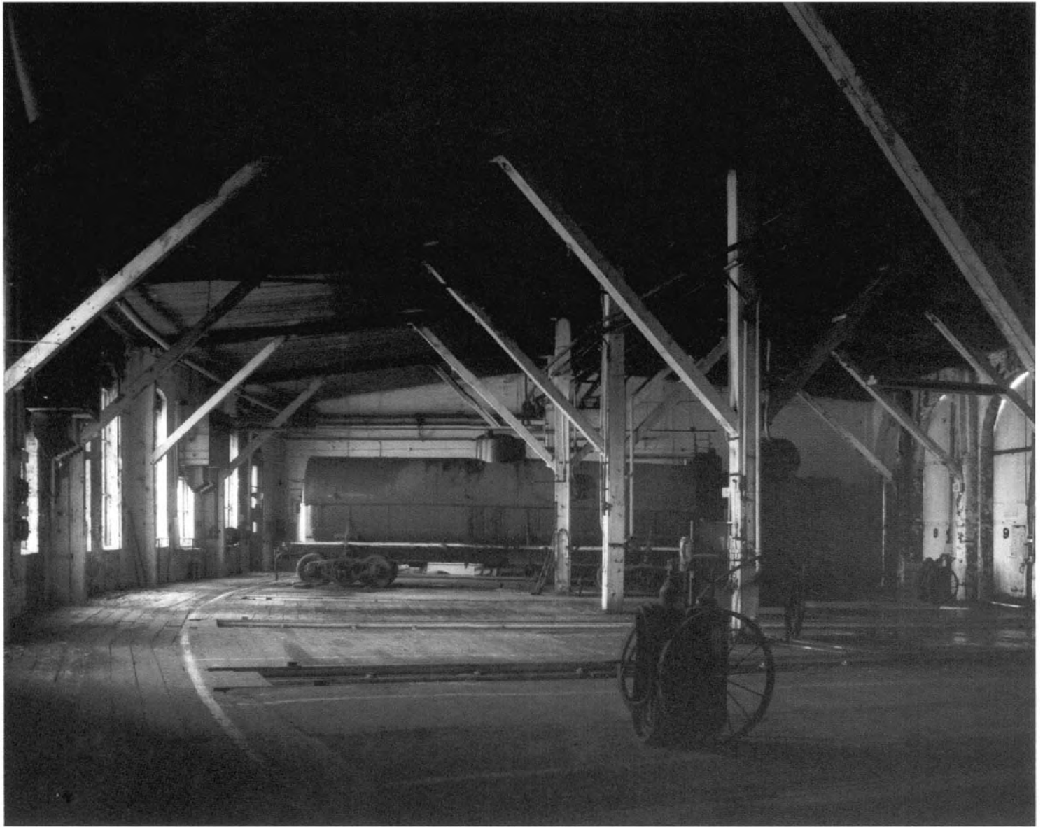
ROUNDHOUSE, SOO LINE SHOREHAM YARDS, NORTHEAST MINNEAPOLIS, 1998
